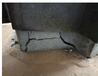
(a) 试件底面裂缝
